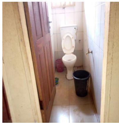
Plate 2: Flush toilet at Uselu market toilet facility
